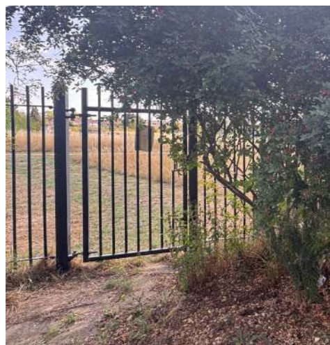
Access gate to Springfields Park
